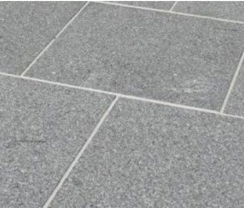
Paving type 1- General paving (grey granite stretcher bond pattern)
