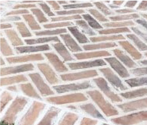
Paving type 2 - Feature paving (herringbone brick pattern)
