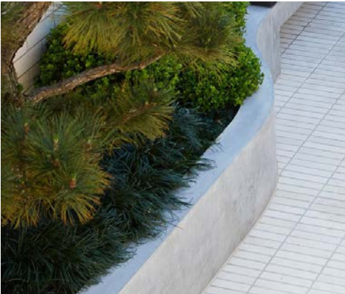
Concrete retaining wall
